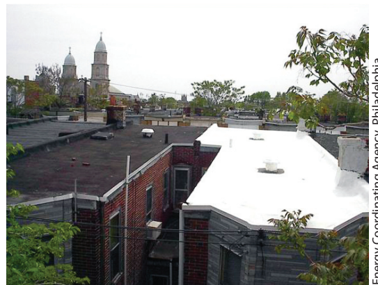
Figure 11: Cool Roofing on Urban Row Homes
