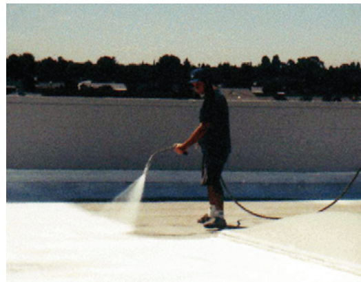
Figure 7: Cool Coating Being Sprayed onto a Rooftop
