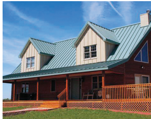
Figure 9: Cool Metal Roofing
