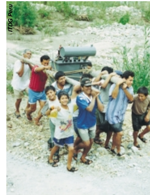
▶ People from the community pull together to transport the step-up transformer to the powerhouse, Peru.
